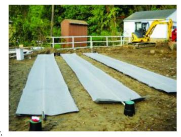
The thin, narrow profile, shallow burial depth and uniform hydraulic loading maximize efficiency of oxygen transfer.
